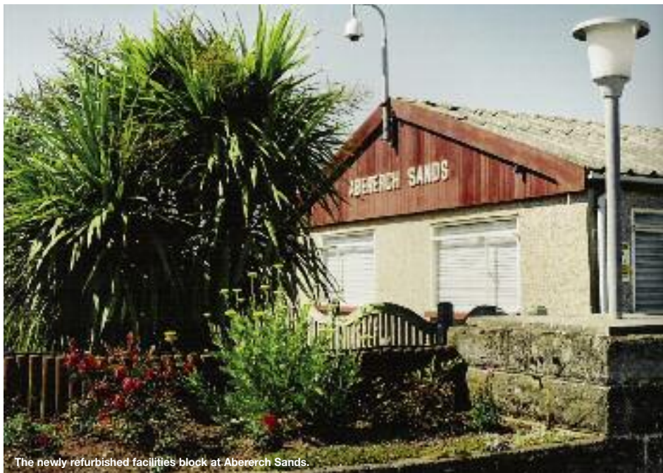
The newly refurbished facilities block at Abererch Sands.
